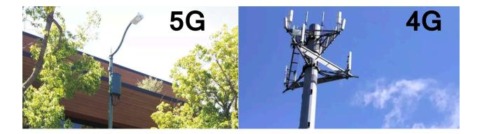
A small cell is essentially just a single node in a 5G network. However, they are probably the most crucial piece of the network, because, without a large amount of them, the information would not be able to relay to its ultimate destination.
